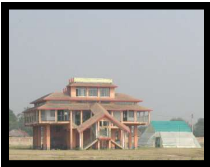
Fig.1c. Hardening unit facility at Women Technology Park, Sagar
